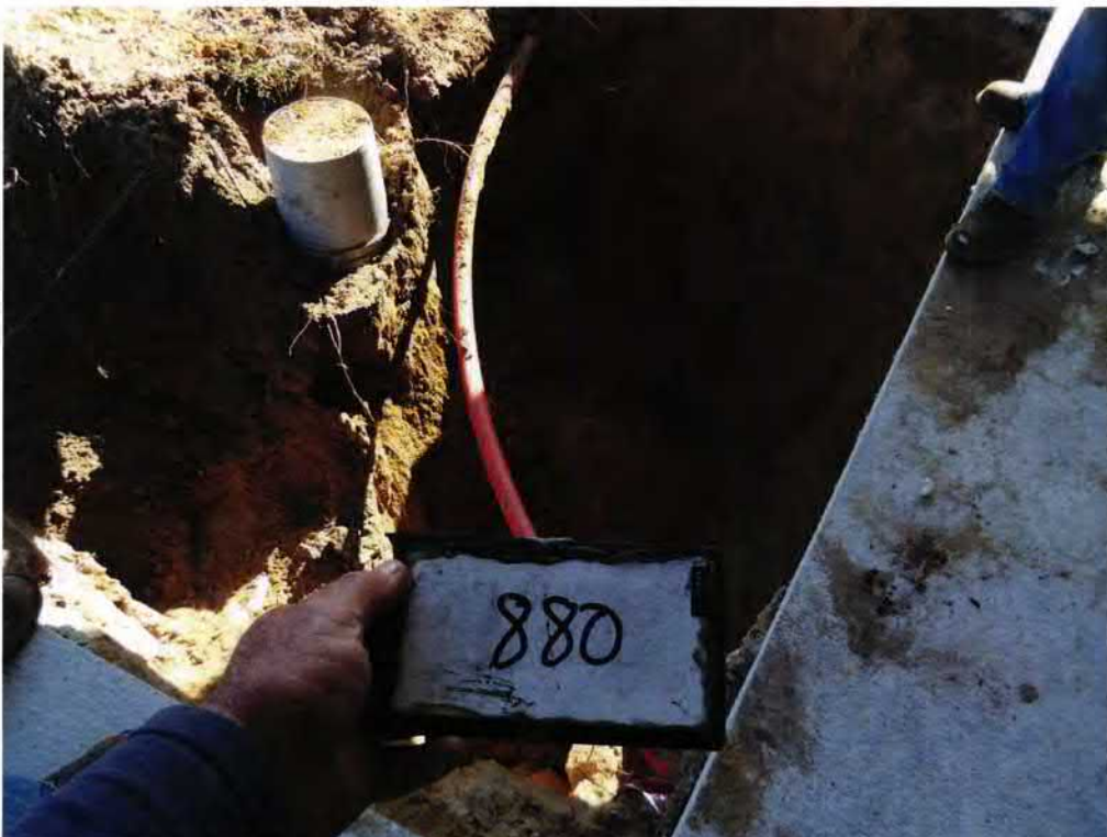
Picture 2: UST 880Cobia excavation.
